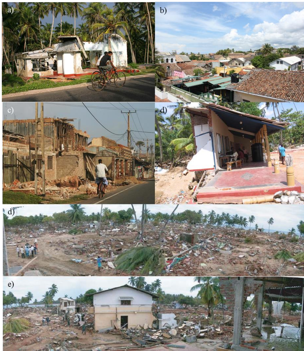
Abb. 3.6: Wohnhäuser in Sri Lanka: a) Galle (Internetquelle 18), b) Galle (Internetquelle 19), c) Galle (Internetquelle 19), d) Peraliya (Borreo, 2005), e) und f) Hambantota (Wijeyewickrema, et al., 2006)
