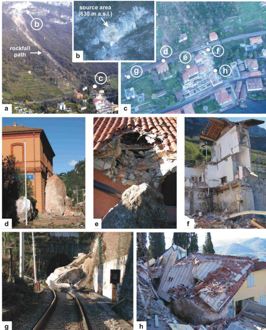
Figure 6.2. The 2004 Fiumelatte rockfall event. (a) NW view of the affected area; (b) source area; (c) impacted area; (d) railway station, damaged by the impact of a 30 m 3 block; (e) roof of building damaged by a 8 m 3 block; (f) three-storey building destroyed by a 96 m 3 block (2 casualties occurred here); (g) damaged railway section; (h) building downslope of building in (F), severely damaged by the same 96 m 3 block (Agliardi et al., 2009).
